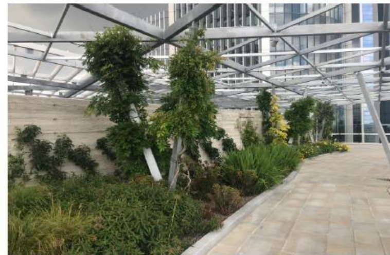
Figure A1.2. Roof gardens are an effective source control element in sustainable drainage systems
