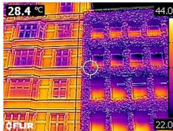
Figure 8. Infra-red image of masonry wall (left) and green wall (right)
